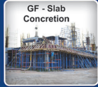
GF - Slab Concrete
